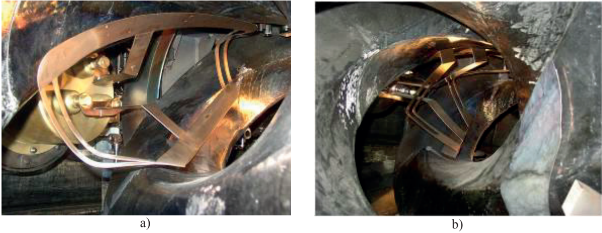
FIG. 34. a) frame antenna, b) three-half-turn antenna installed inside helical coils.
